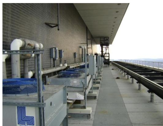
All four sides of the overhang were shot with the IR as was the interior ceiling of the electrical and mechanical floor. Some sections of this floor were open on the side for ventilation. The restaurant sits on top of this overhang and the mechanical floor. There are great views of the city all around the building from the restaurant floor but a cold air problem had invaded this floor level causing the comfort and cost issues. Two main issues were discovered utilizing the infrared survey.
